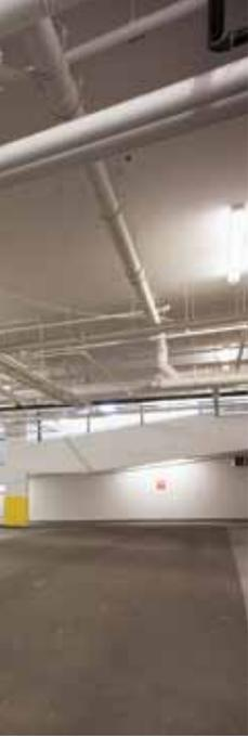
Colour palettes, construction materials and specifications differentiate this property from any other in Alberta. Precast was chosen for its resilience and inherent fire resistance - both being key requirements for this property. The interior uses long-span concrete hollowcore floor slabs supported by precast concrete shearwalls.
